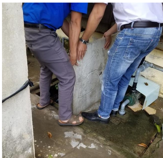
Figure 32: Employee in Sandals Lifting Heavy Concrete Cover
