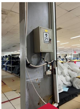
Figure 22: Ungrounded Outlet in Production Area
