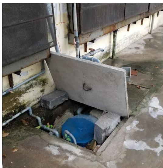
Figure 31: Heavy Concrete Cover for Evaporative Cooling System Sump
