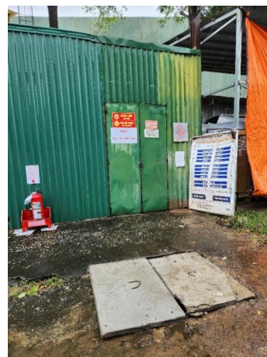
Figure 7: Dilapidated Cover Holes
