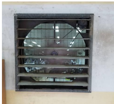
Figure 14: Unguarded Fan Blades inside Dampers
