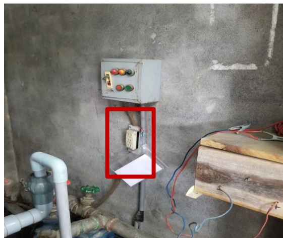
Figures 20 and 21: Ungrounded Electrical Outlet in Fire Pump Room
