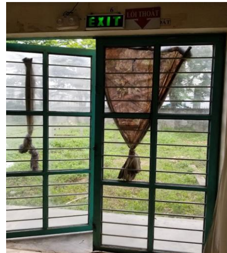
Figure 3: Exit Door 'Pinned' Partially Open
