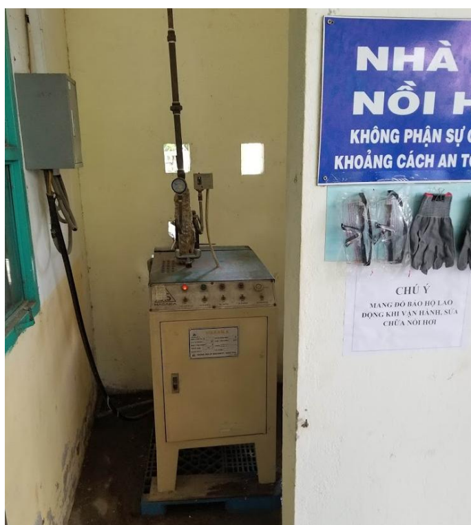
Figure 12: Steam Compressor with Only Safety Glasses and Gloves Provided for PPE
