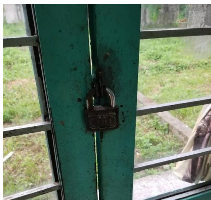
Figure 2: Locked Exit Door
