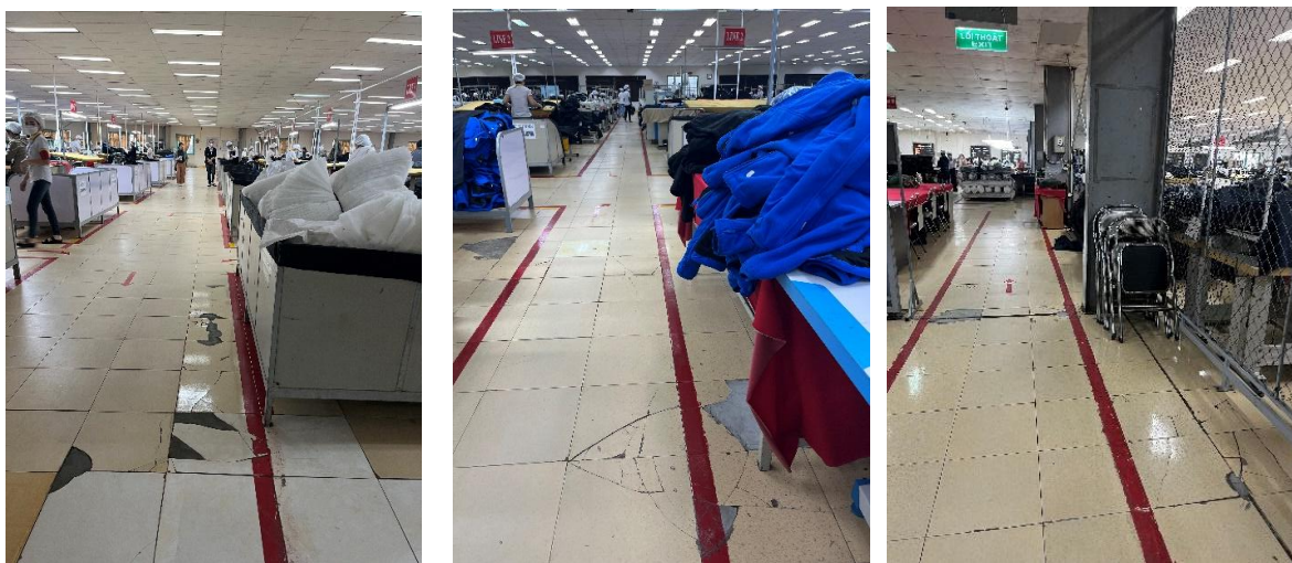
Figures 4, 5, 6: Broken Flooring at Walkways
