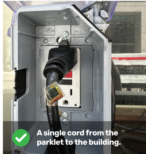
✓ A single cord plugged directly into electrical outlet is easy to unplug in case of emergency.
