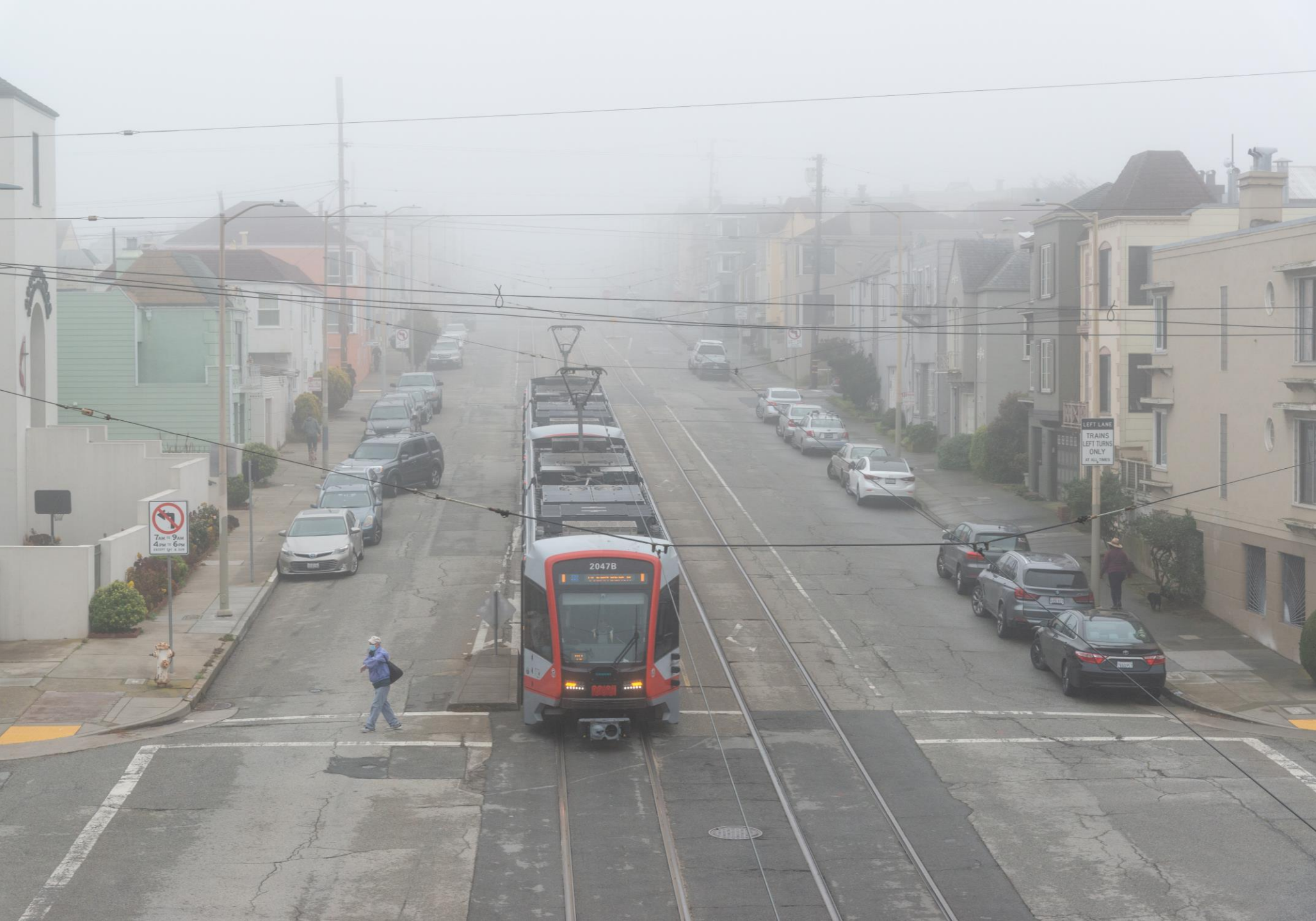
Overhead View of N Judah Stop Before Improvements | March 15, 2022
