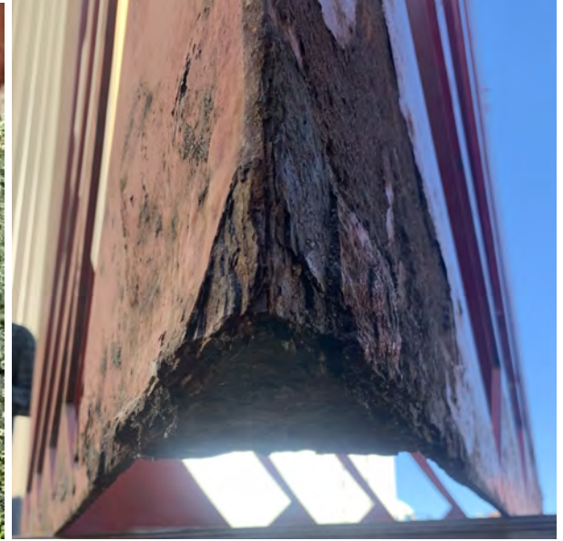
Deteriorated Corner Block 3 Showing Paint Failure and Delaminating Metal (Left) Deteriorated Corner from Underside Showing Loss of Material (Right)
