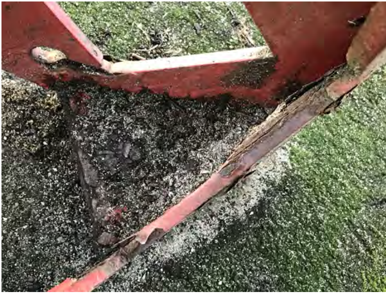
Deteriorated Corner Block 3 Showing Paint Failure and Delaminating Metal (Left) Deteriorated Corner from Underside Showing Loss of Material (Right)
