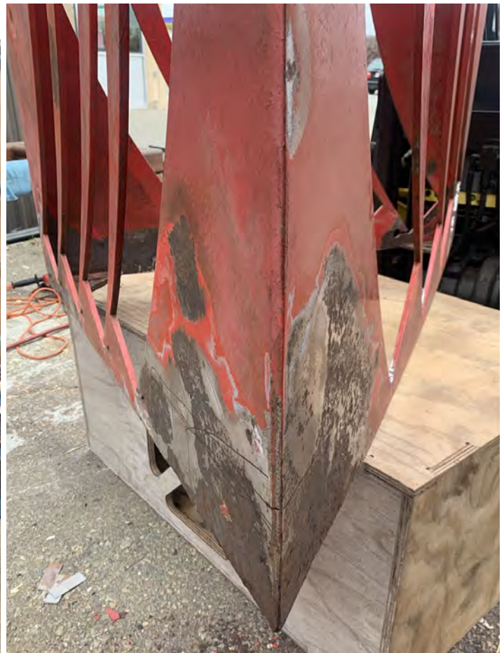
Signature Side After Grinding. Areas Marked with Sharpie Were Replaced (Left) Detail of Corner with Ground Metal (Right)
