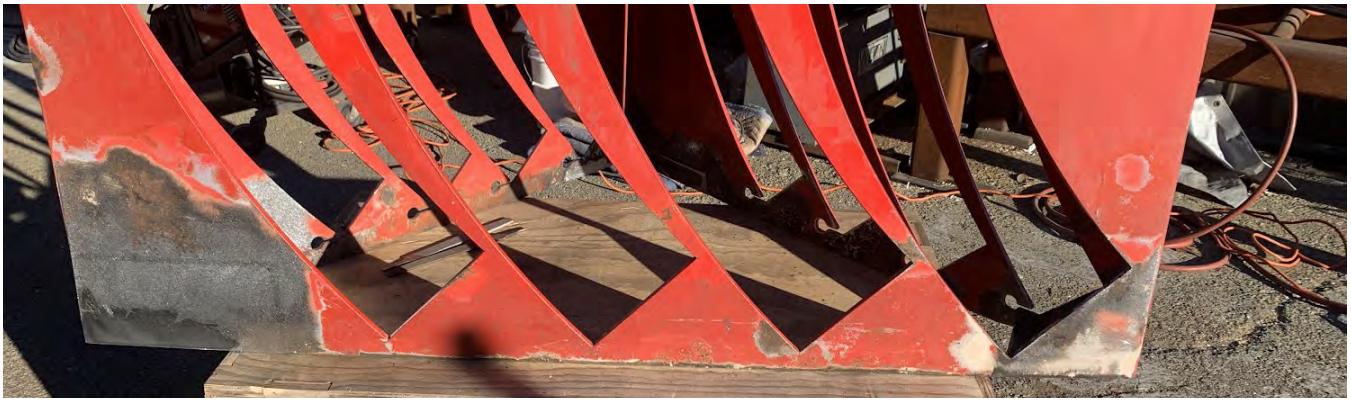
Detail of Long Side After Metal Repairs
