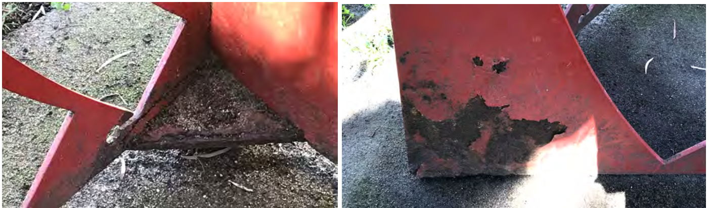
Detail of Corner Plate 1 (Left) Showing Organic Material, Corrosion, Blistering Paint and that the Bolt Head has Corroded Off Exterior Lower Corner 2 (Right) with Blistering Paint, Losses and Corroded Substrate
