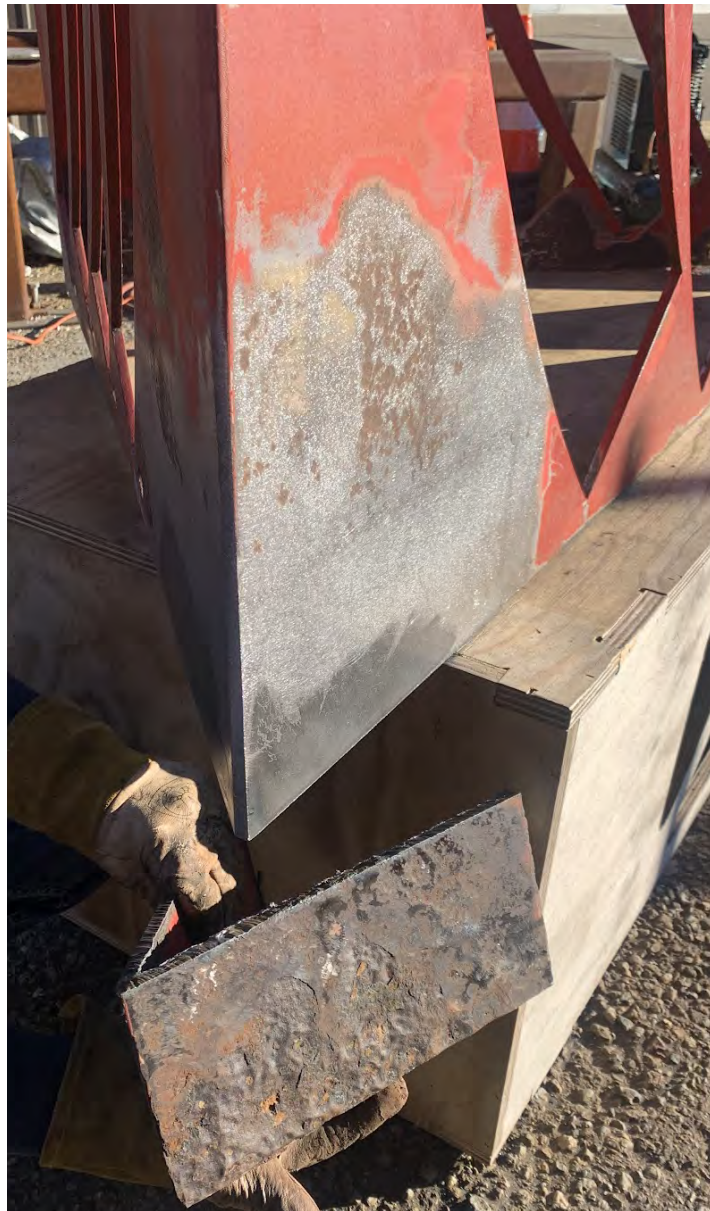
Detail View Showing Replaced Corner between Long Side and Short Side Without Signature
