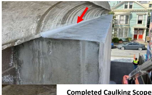
Completed Caulking Scopes
