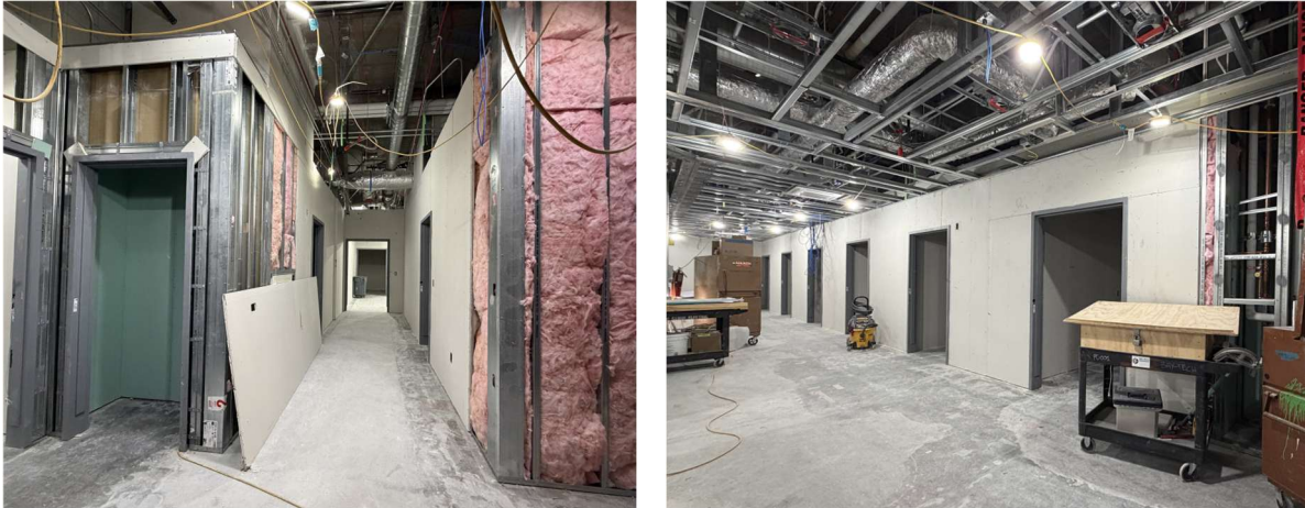
Circulation Area and Seclusion Rooms
