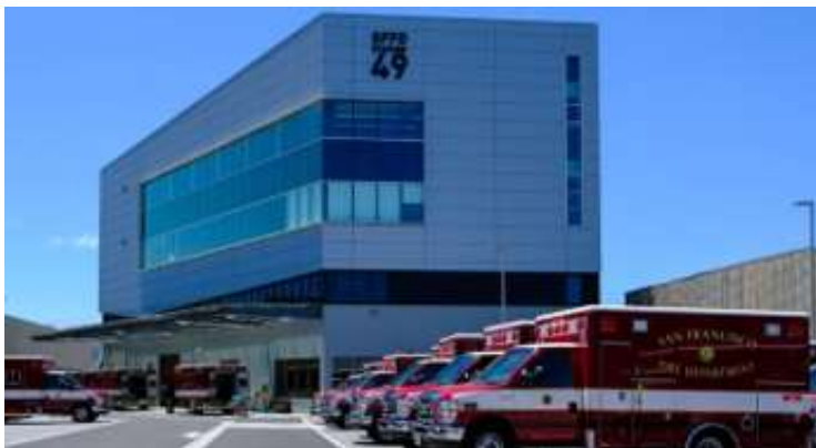
Ambulance Deployment Facility
