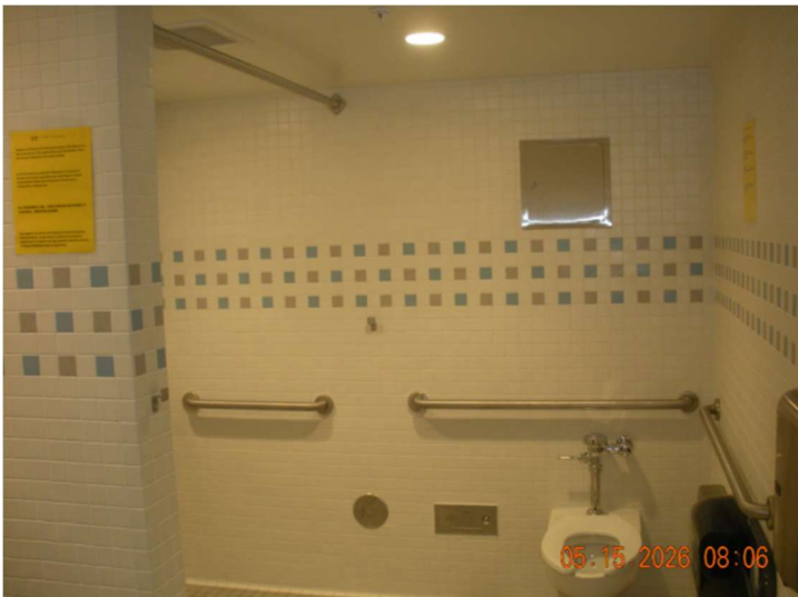
1 st Floor All-Gender Restroom/Shower (Public-Use)
