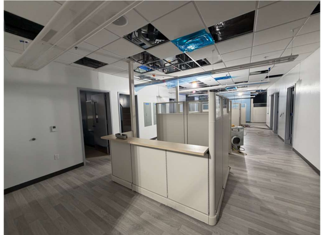
Furniture Installation at Admin area
