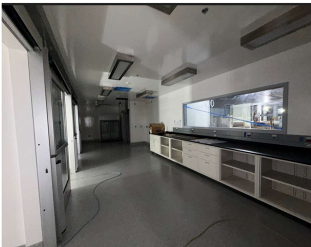
Completed BSL-3 Lab Wall Finishes
