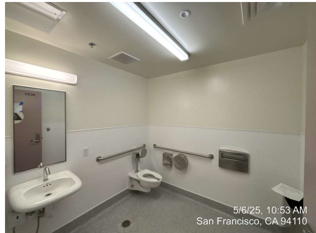
Ward 3A/3C Restroom – Complete
