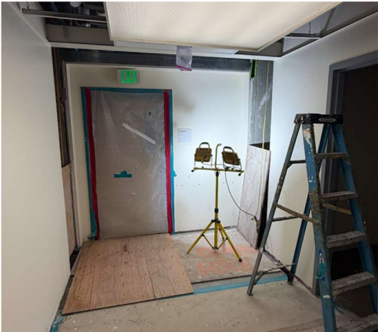
L5 Interior finishes and future 25" Seismic Expansion Cover
