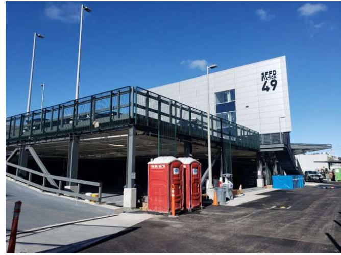
View of backside of the new SFFD Station 49 and upper garage deck.
