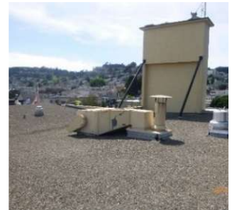
Fire Station Hose Tower
