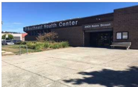
Existing SE Health Center
