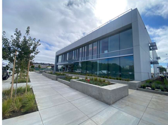
S/W View of Building
