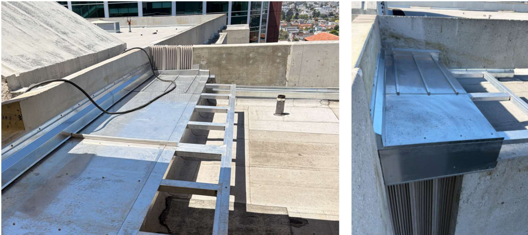
Roof 25" Seismic Expansion Cover
