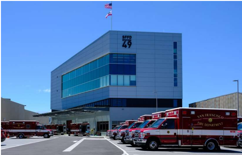
Front of New SFFD Station 49
