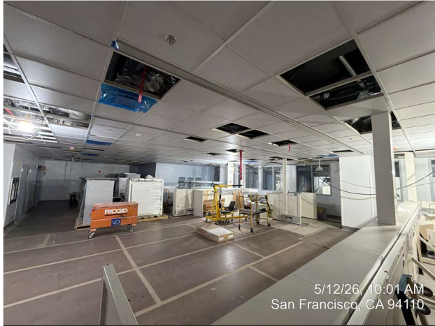
BSL-2 Lab casework installation and Ceiling Close up
