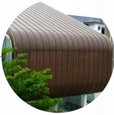
KYNAR FINISHED ALUM. STANDING SEAM ROOFING
