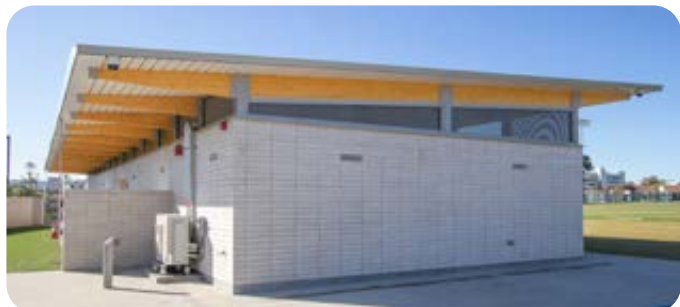
4X16 STACK BOND - BURNISHED FACE CMU BLOCK
