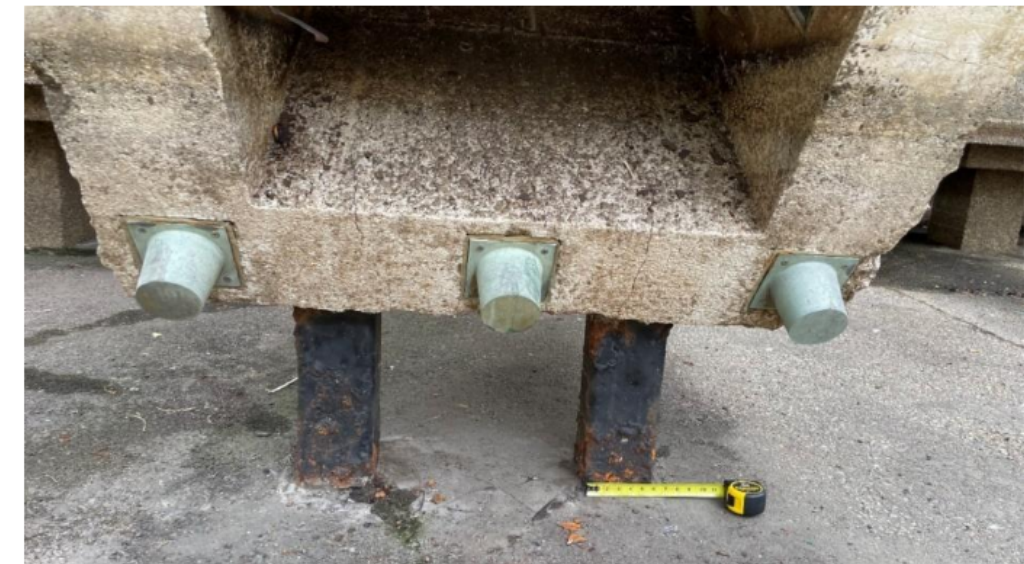
Figure 8: Vaillancourt Fountain - Corroded Steel Tubes and Spalled and Cracked Concrete
