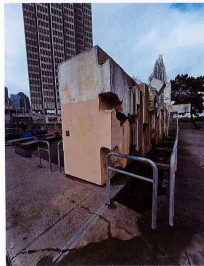
Photo 4. Rear wall – no reinforcing steel was found.
