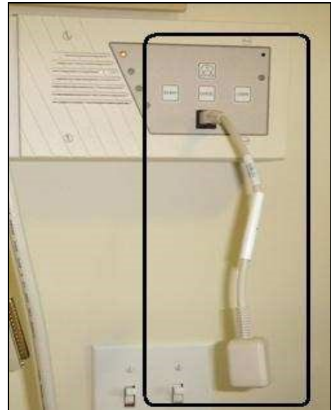
CIRCLED AREA SHOWS THE SOCKET FROM CONNECTING CORD ATTACHED TO THE NURSE CALL PANEL.
