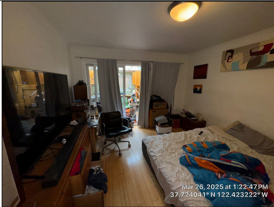
Figure 5. Rear right second-floor bedroom. Its only connection to the rear is an interior sliding glass door (rear of room), opening not to the exterior but into an enclosed former porch.
