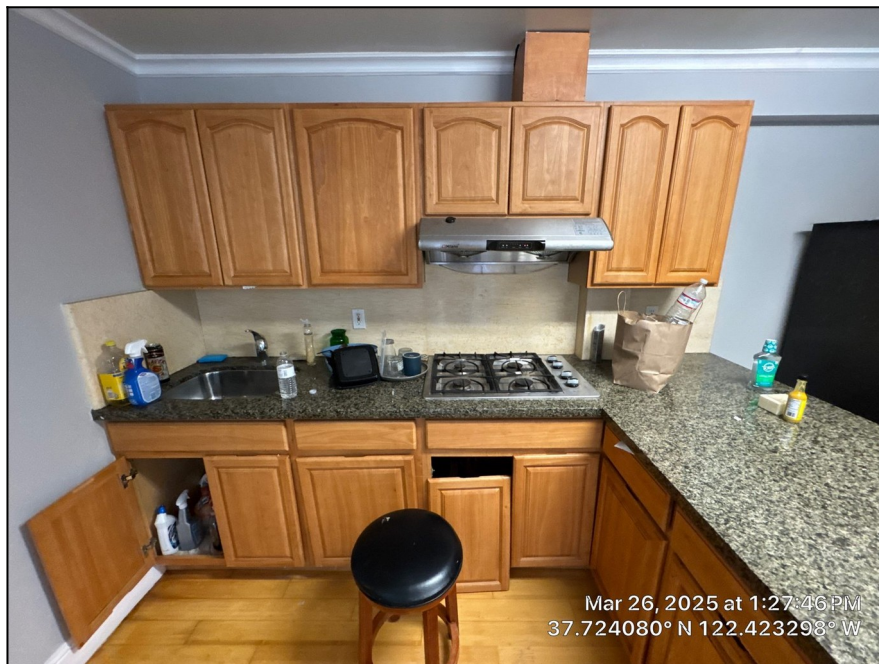
Figure 4. The same unpermitted ground-floor kitchen from a second angle, showing the gas cooktop and full cabinetry of the unauthorized dwelling unit.
