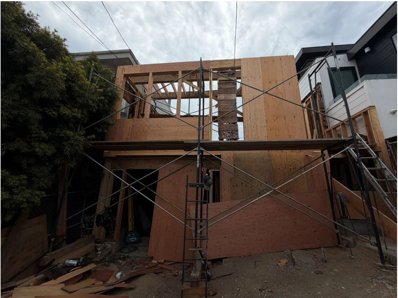
Figure 1 of 2. Photo showing the front façade with original framing removed.
