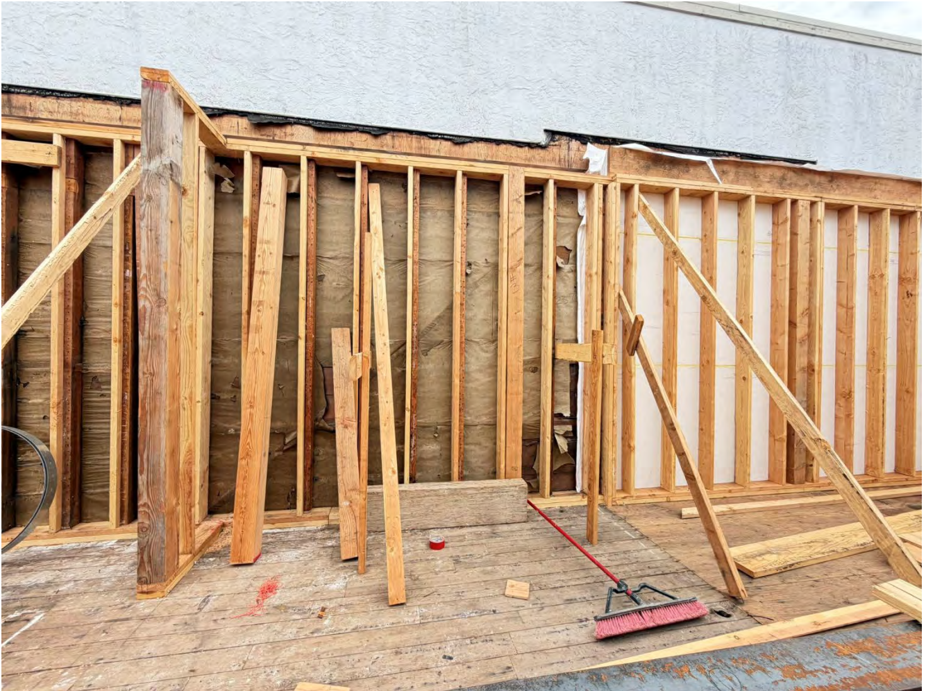
Figure 2 of 2. Photo showing all new side wall framing above the 2 nd floor.
