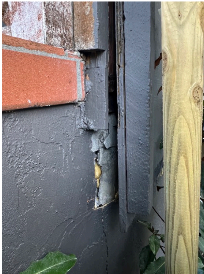
Detached sheathing and cracked foundation
