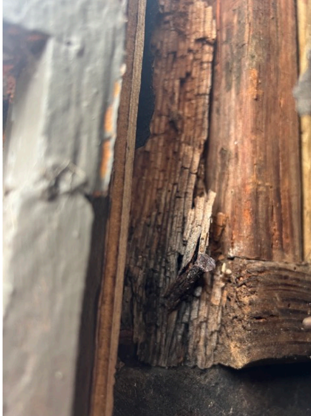
Damage behind detaching sheathing
