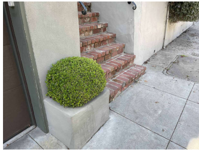
DETAIL OF ENCROACHMENT AT 100 ALPINE TERRACE.
