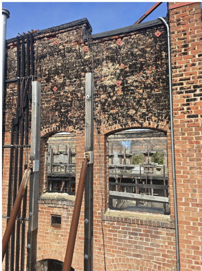
Unbraced “parapets” 02/04/2025
