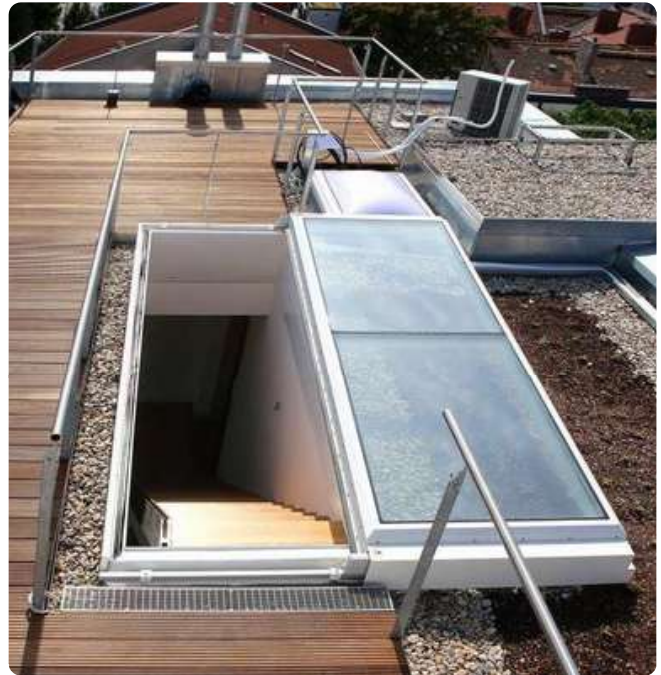
A roof hatch that would not require public notice. (iStock)
