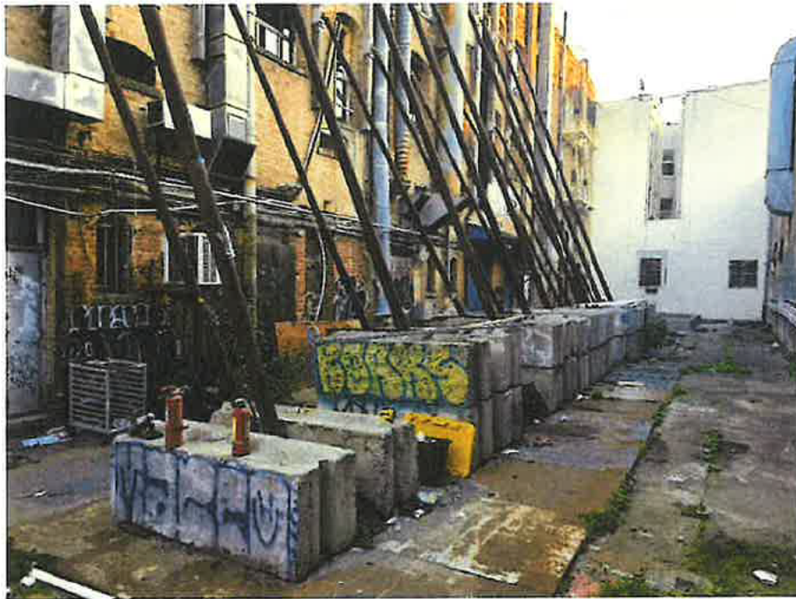
Rear Yard Out-of-Plane Wall Bracing System
