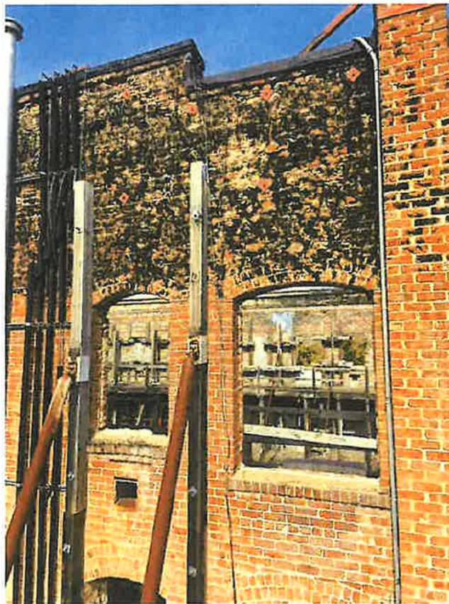
Unbraced "parapets" 02/04/2025
