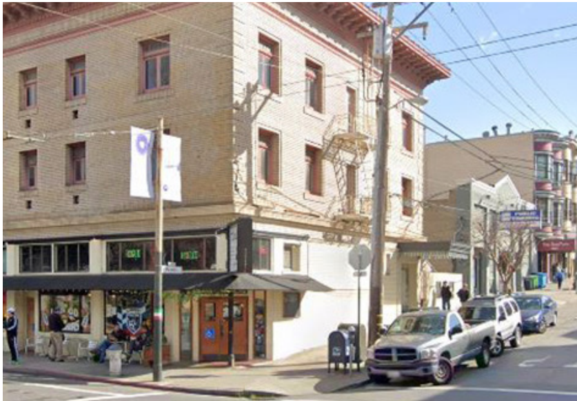
Material of previous building before fire.
