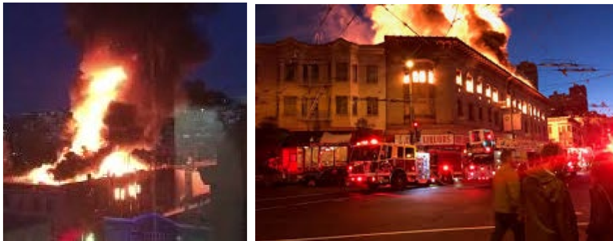
Images of the subject building ablaze, March 2018
