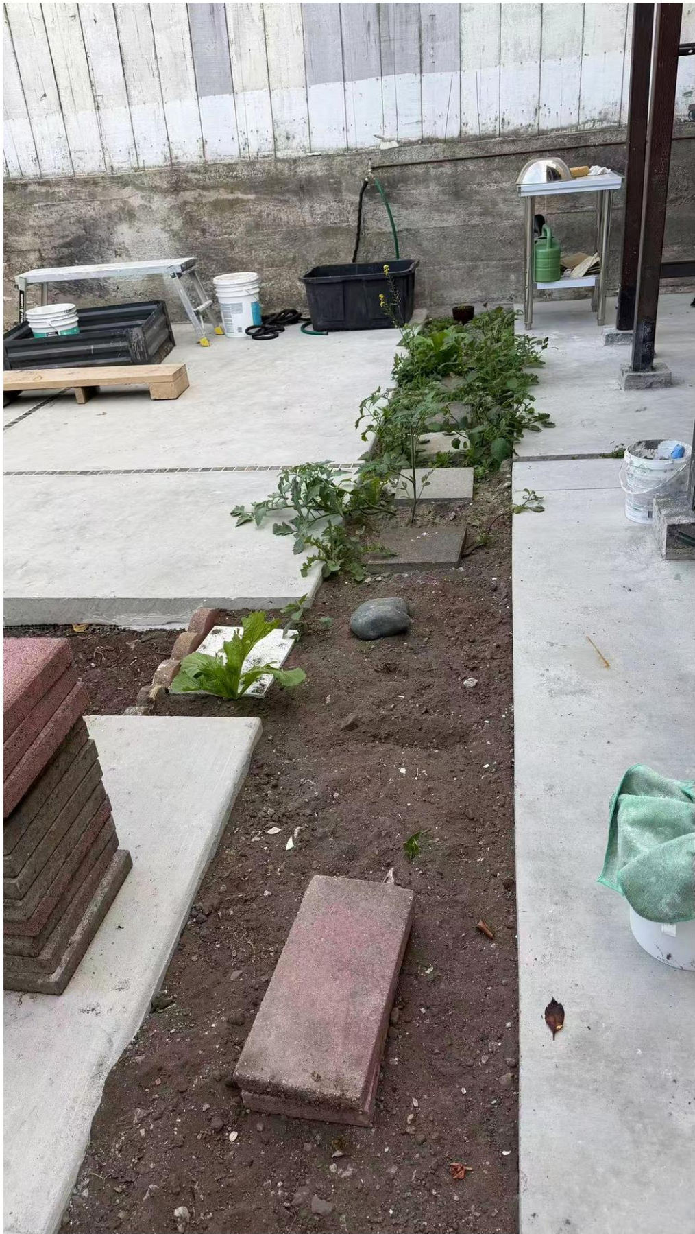
Current rear-yard condition (October 2026): planted drainage strip between subdivided concrete sections.
