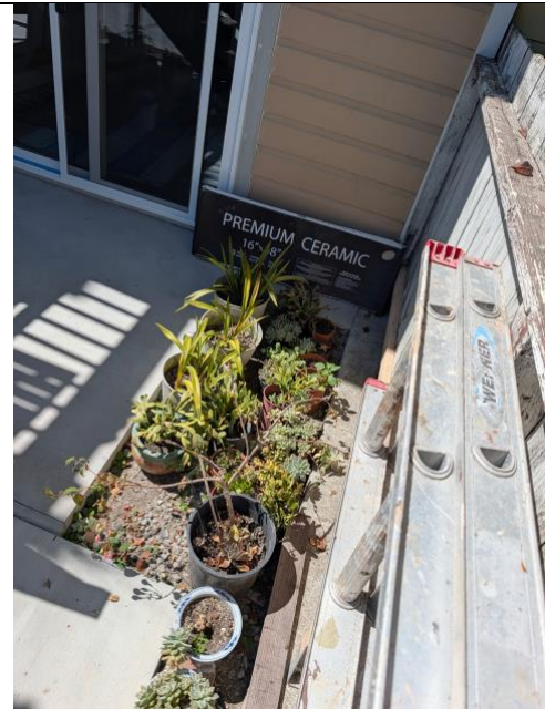
Current condition. Widened but same termination point. Yard and RW grade are at the same elevation.
