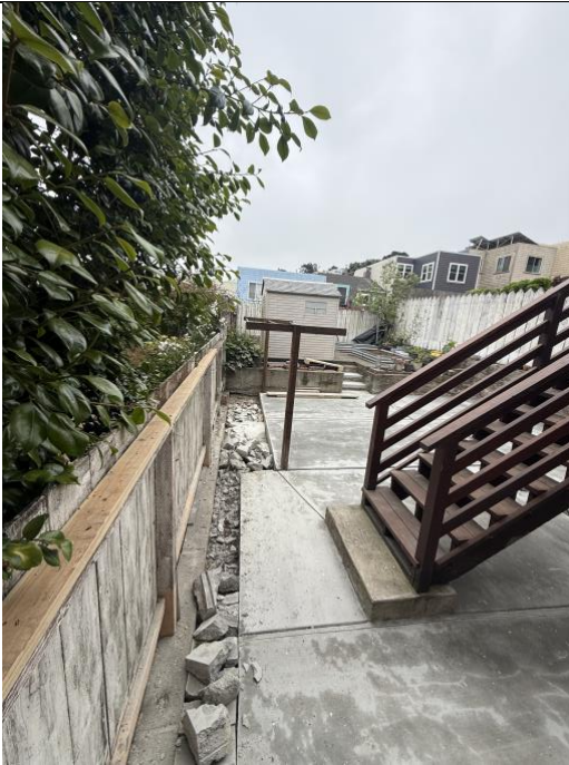
Soil strip sawcut after the correction along lower retaining wall.
