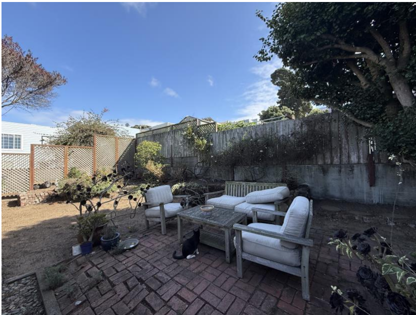
Two tier retaining wall as seen from Appellant's rear yard. Concrete slurry whitening/bleaching visible.
