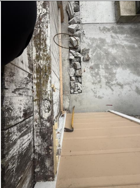
Soil strip sawcut termination point.
