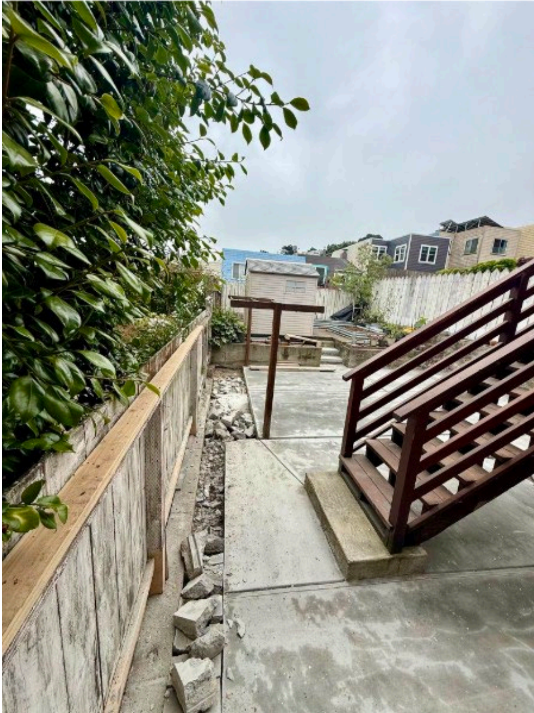
Exhibit 1: Saw-Cut Concrete After Initial Pour
