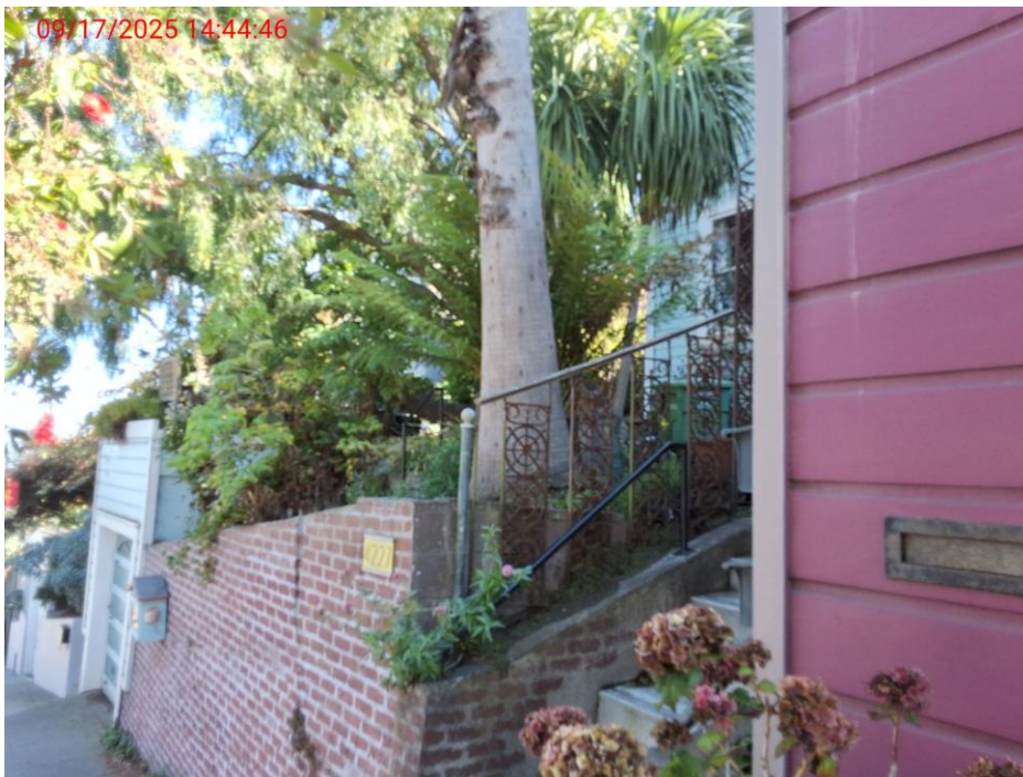
Exhibit 3. Photo of the retaining wall at 4227 26th Street.
