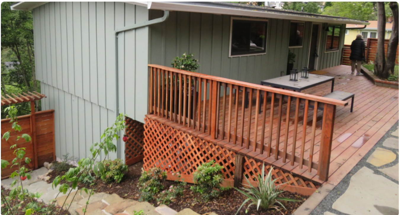
Rear elevated deck on slope. (Fabrice Florin, Flickr, CC BY 2.0)
