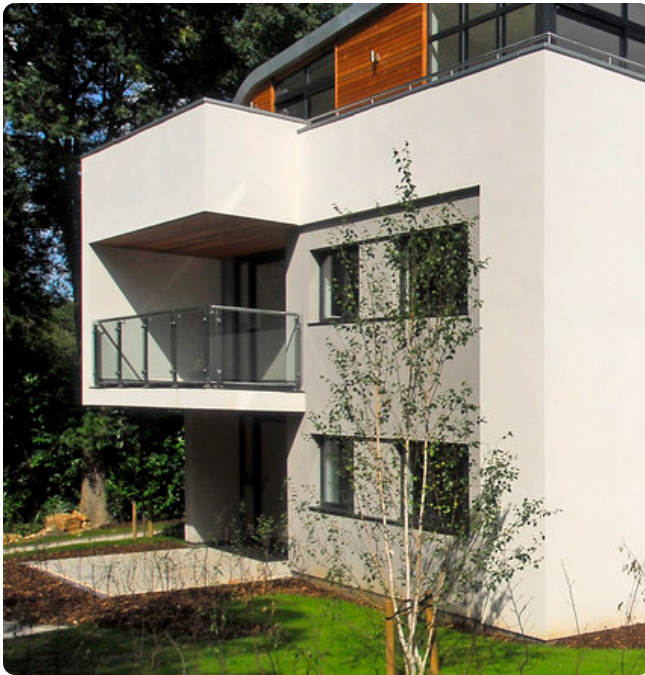
Cantilevered decks. (Darrel Godliman, Flickr, CC BY 2.0))
