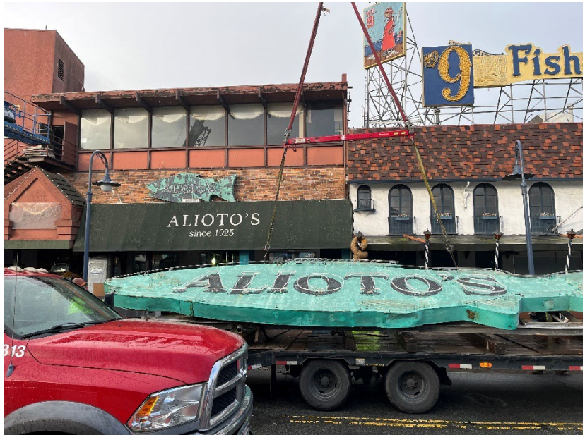
Figure 3: Taylor Street Seawall earthquake stabilization project.
