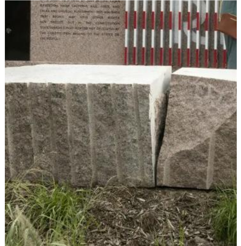
FLAMED TOP + QUARRY DRILL FINISH
