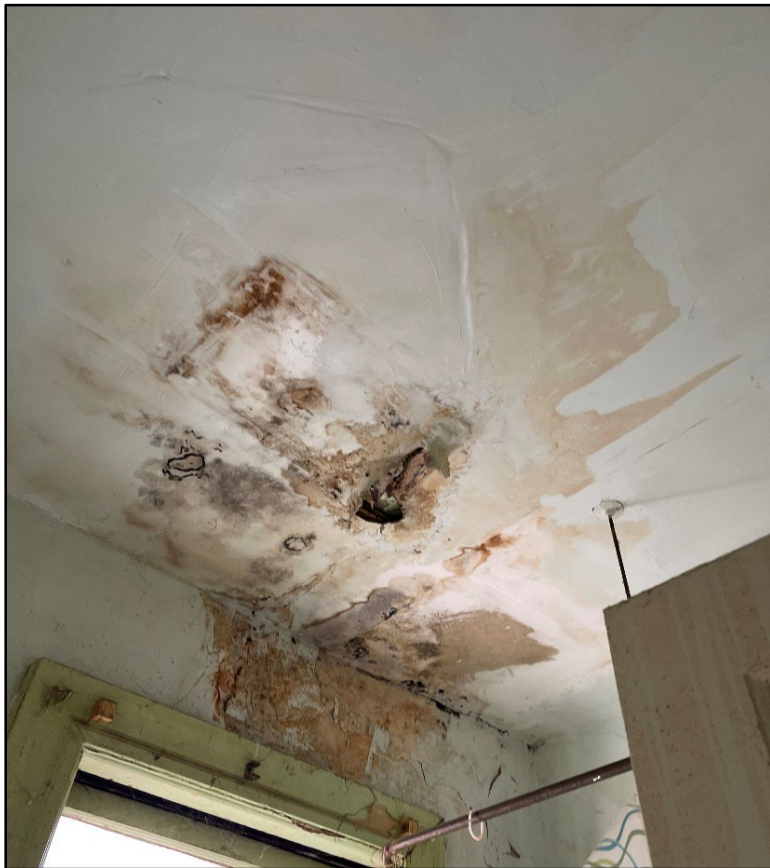
Field inspection photos: Severe water damage
