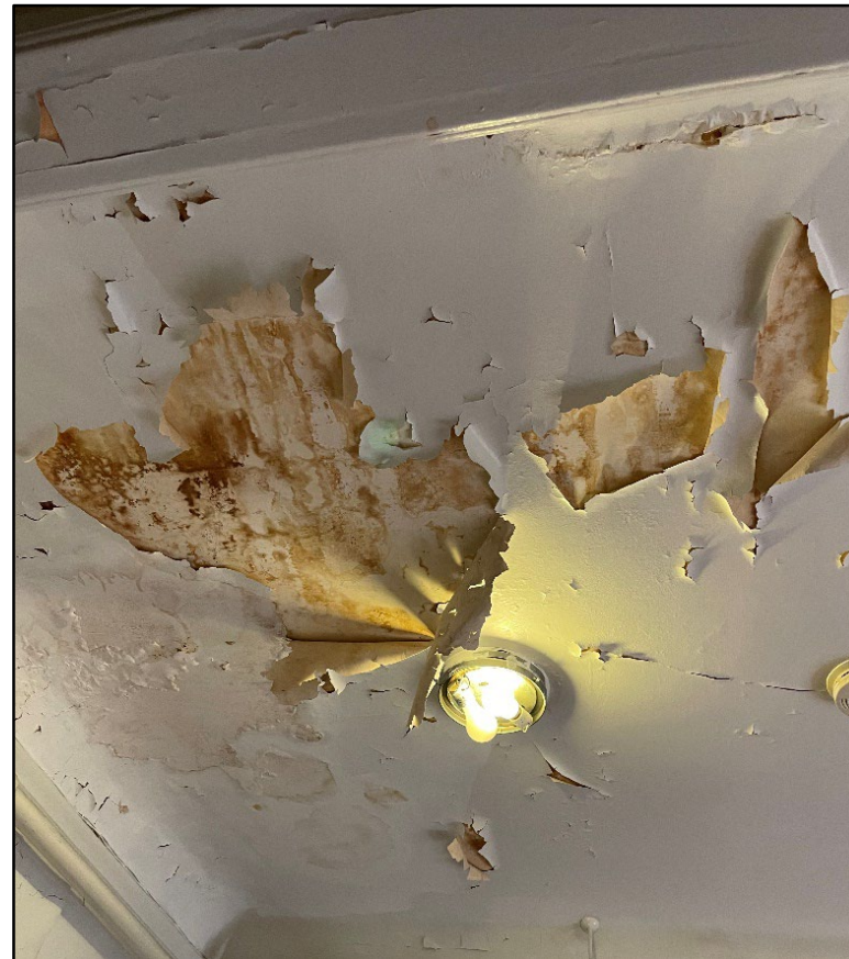
Field inspection photos: Severe water damage
