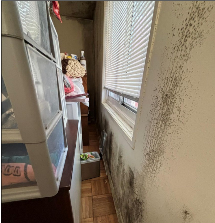
Photos from the field: Black mold and water intrusion
