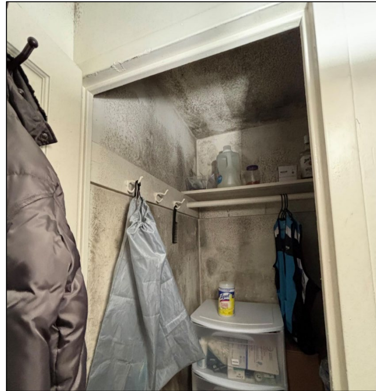
Photos from the field: Black mold and water intrusion
