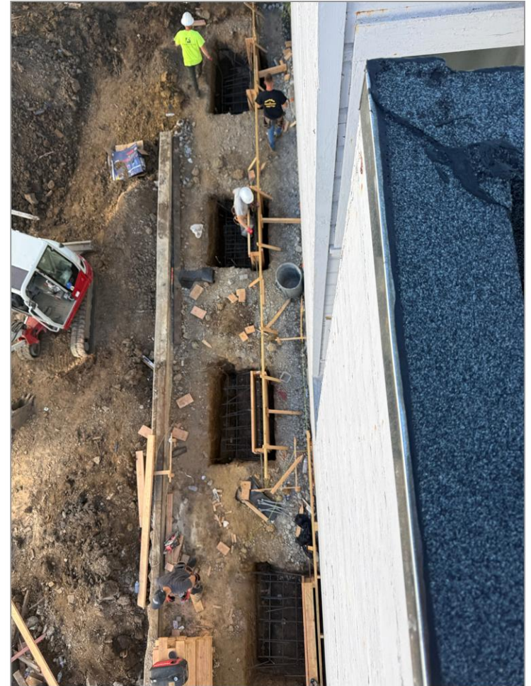
Mar 20, 2026, 10:14 AM, from our window: new footings and rebar along our wall.
