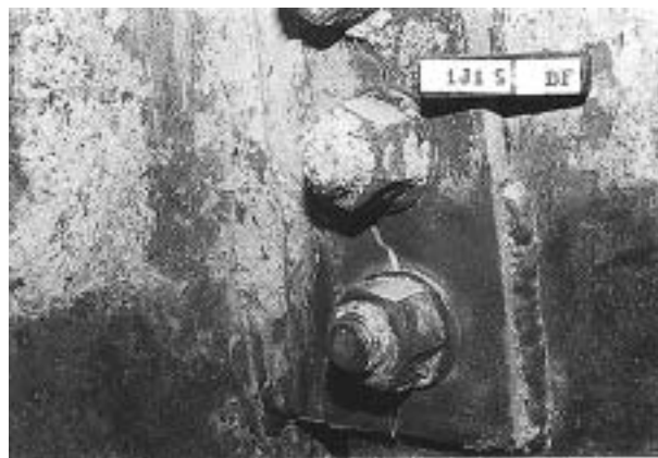
Figure 1-5 Vertical Fracture through Beam Shear Plate Connection
