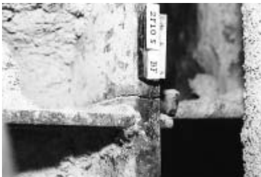
a. Fractures through Column Flange
