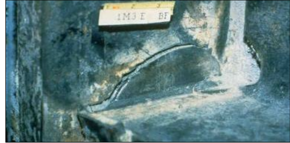
A cracked weld identified after the Northridge earthquake in 1994
