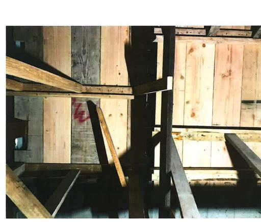
Shoring and forms for replacing section of retaining wall next to and below garage floor.
