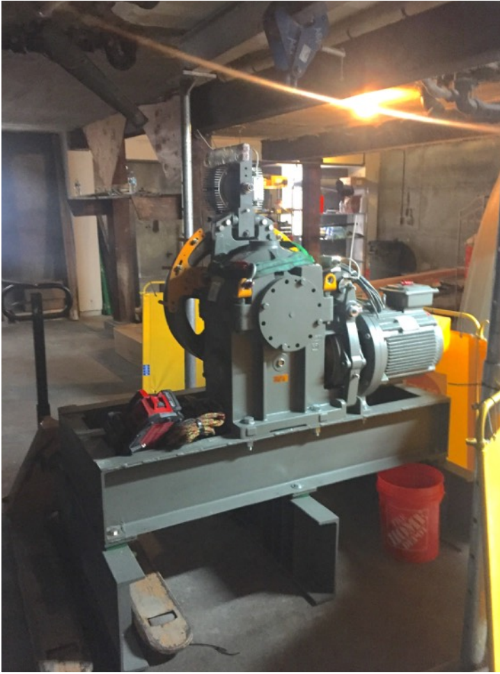
New Motor on site, February 23, 2021
