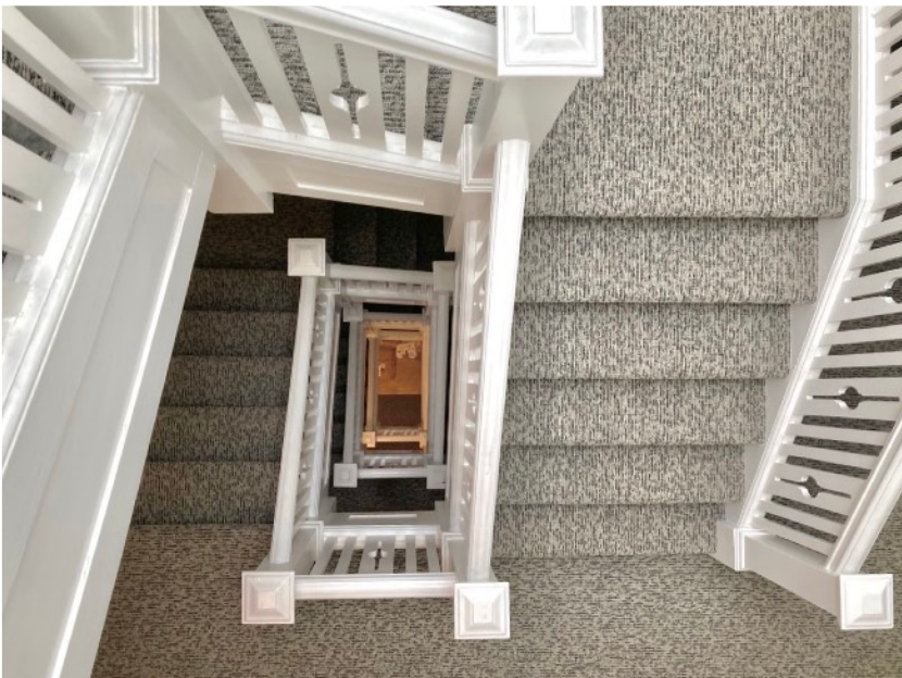
Existing 4-Story Common Stairwell - 2960 Polk Street
