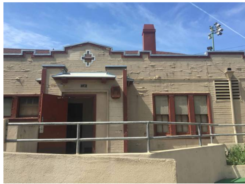
8 (E) CLUBHOUSE EXTERIOR - EAST - PHOTO 1
