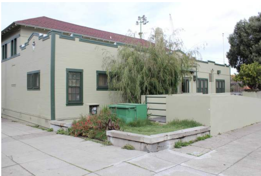
9 (E) CLUBHOUSE EXTERIOR - EAST PHOTO 2
