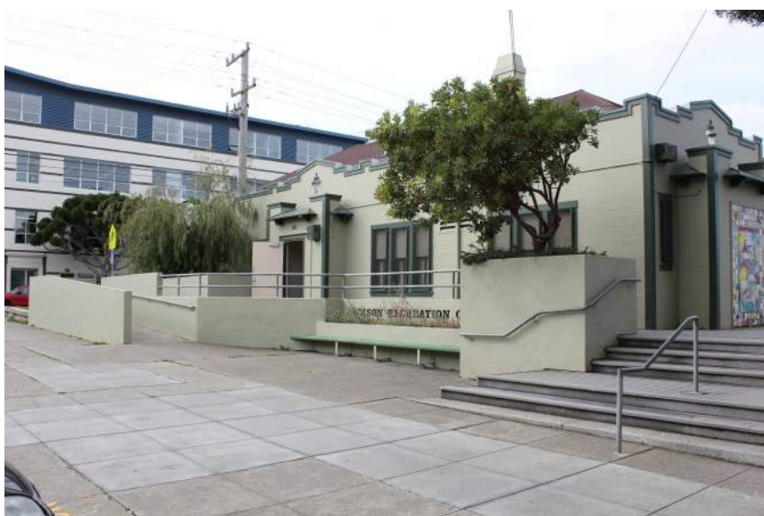
11 (E) CLUBHOUSE EXTERIOR - EAST PHOTO 3
