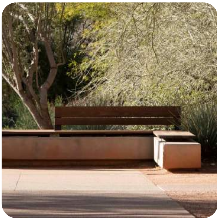
CAST IN PLACE CONCRETE WALLS WITH INTEGRAL COLOR
