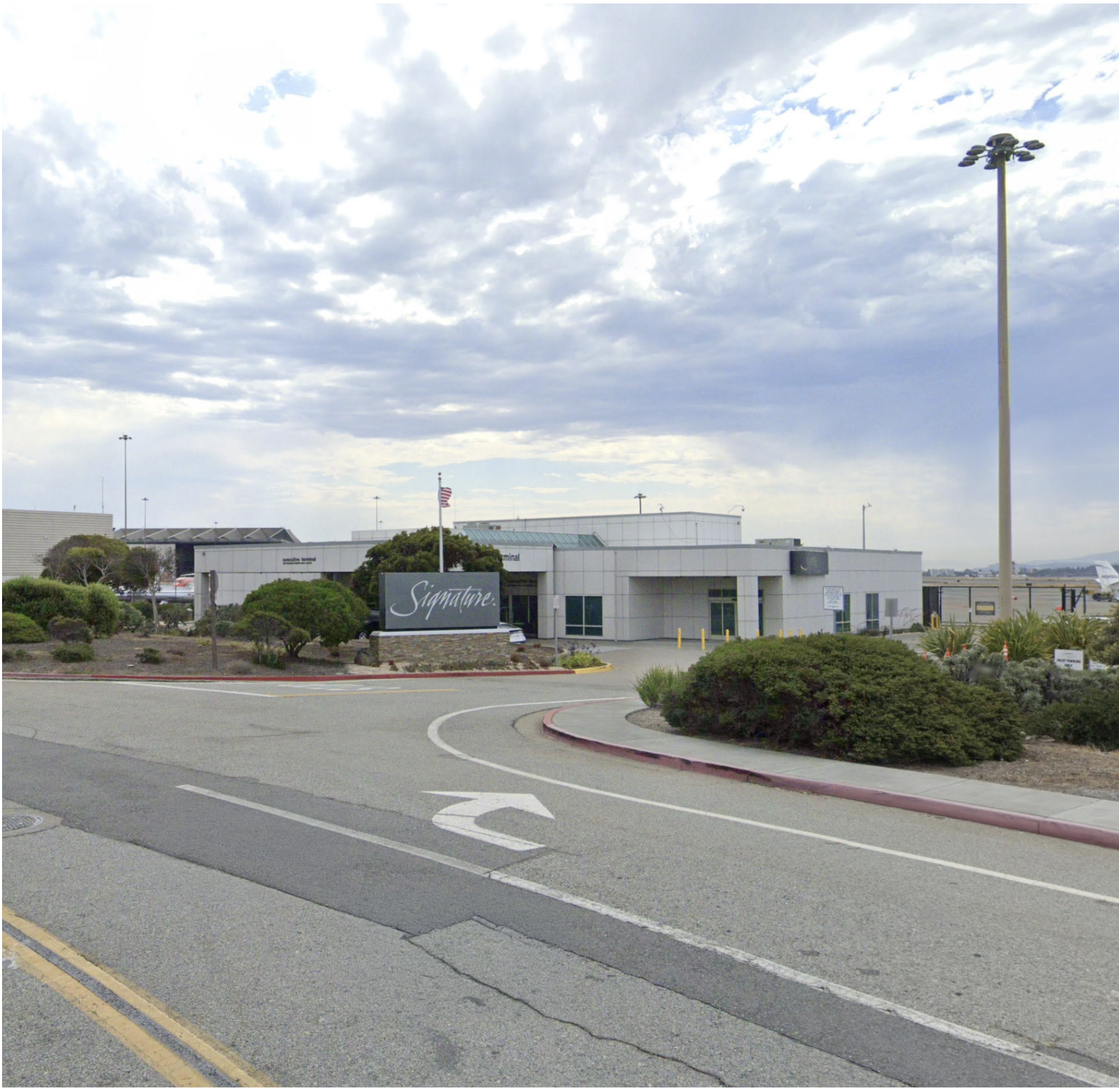
EXISTING TERMINAL | NORTHWEST
