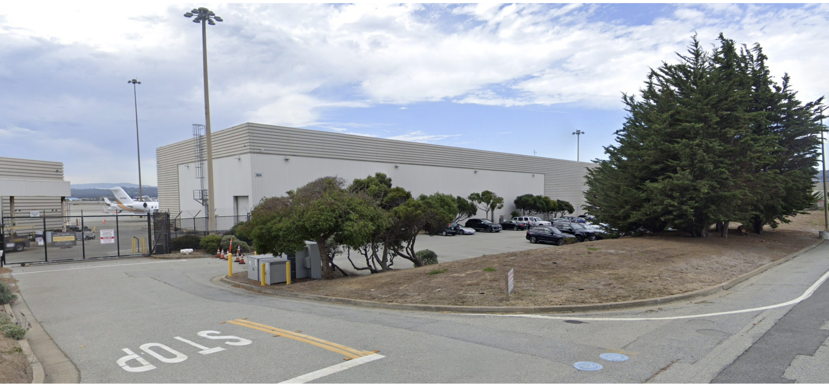
HANGAR A | NORTHEAST
