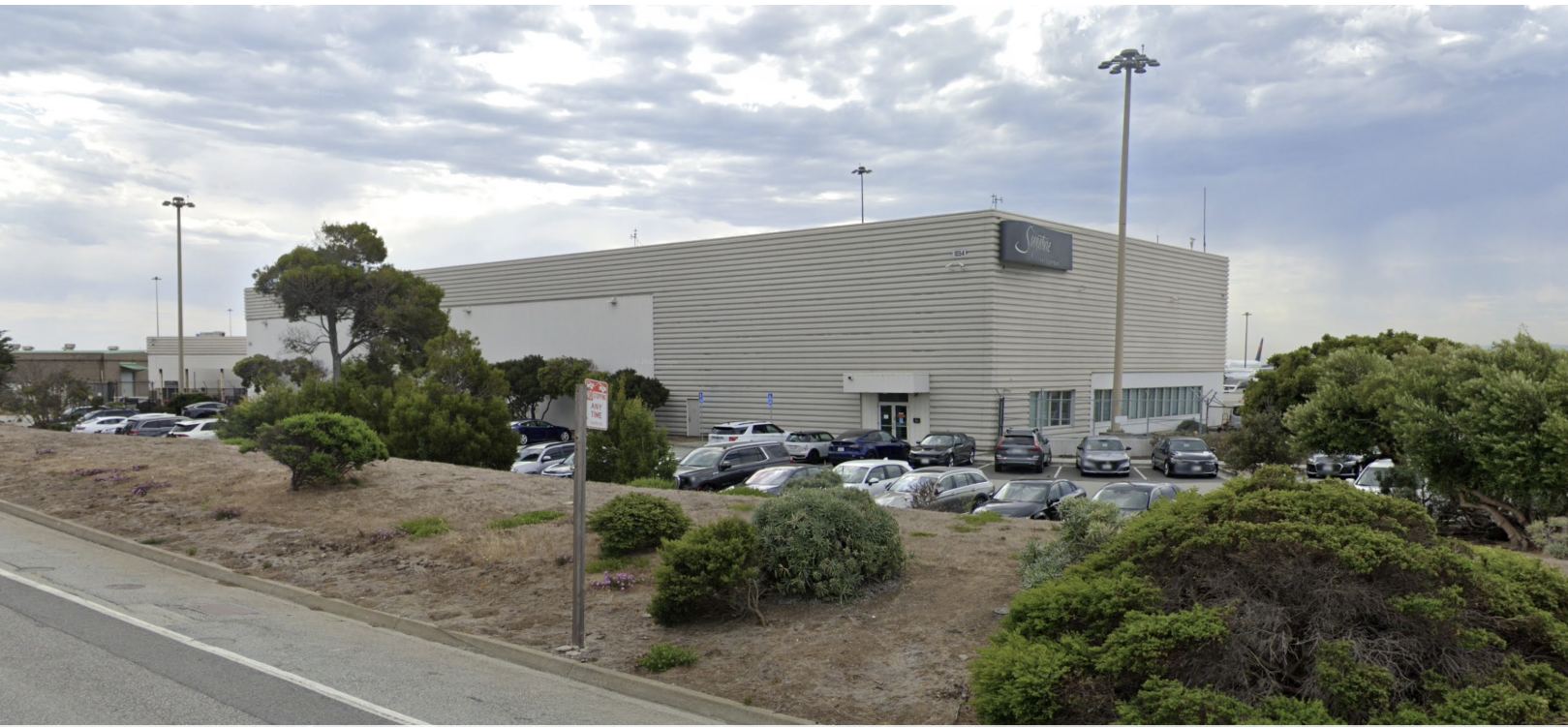
HANGAR A | NORTHWEST
