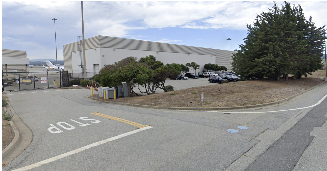
Hangar A - Northeast
