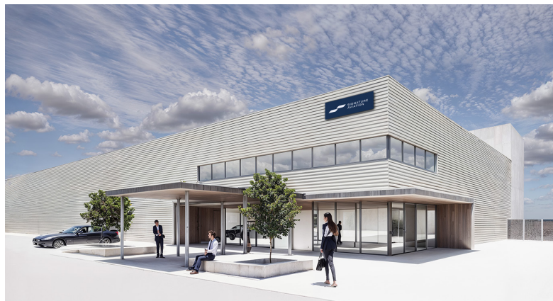
2. TEMPORARY FACILITY - CORNER VIEW
