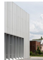
TEXTURED CEMENTITIOUS CLADDING METAL FINS
