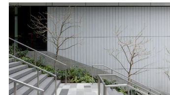
TEXTURED CEMENTITIOUS CLADDING METAL FINS
