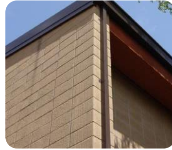
5 EXISTING CONCRETE MASONRY UNITS
