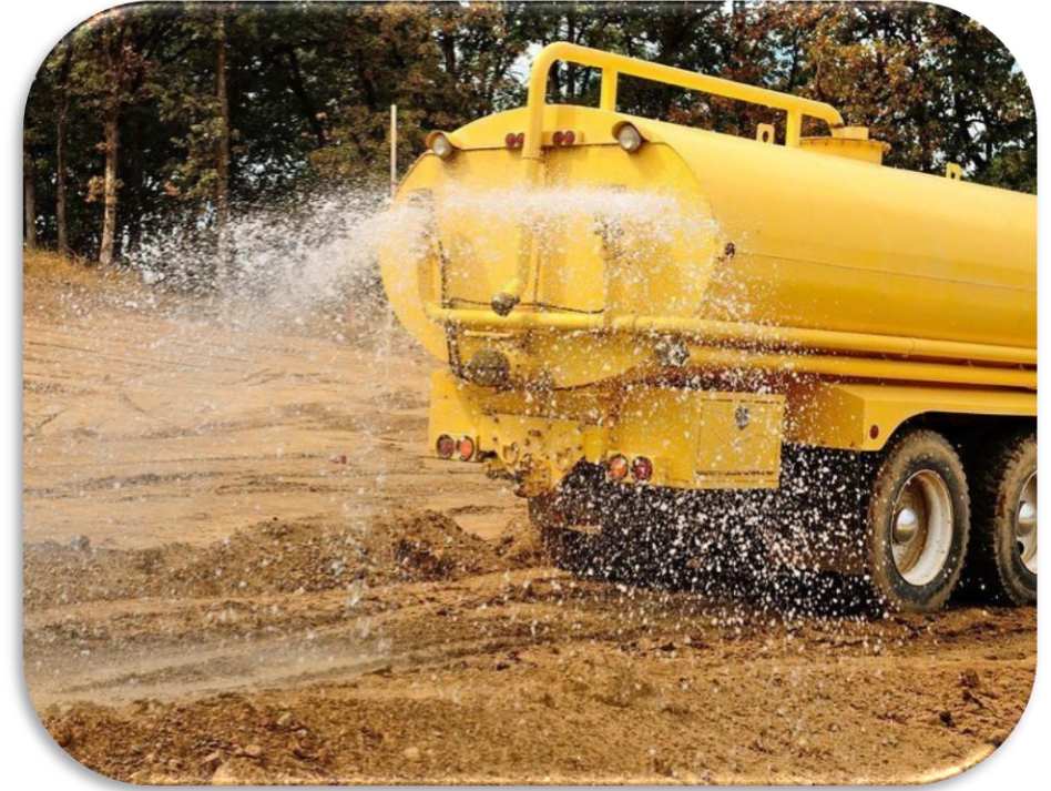
Photo Description: Water application for dust control.
