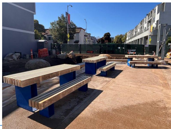
Buchanan in construction
