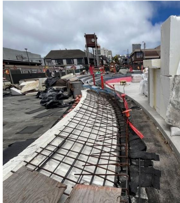
Working on the pagoda and plaza
