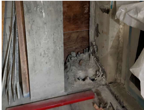
L7 25" Seismic Expansion Joint Wall, Column, and Slab Demo
