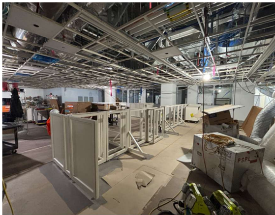
Ceiling Grid Installation and Lab casework at BSL-2
