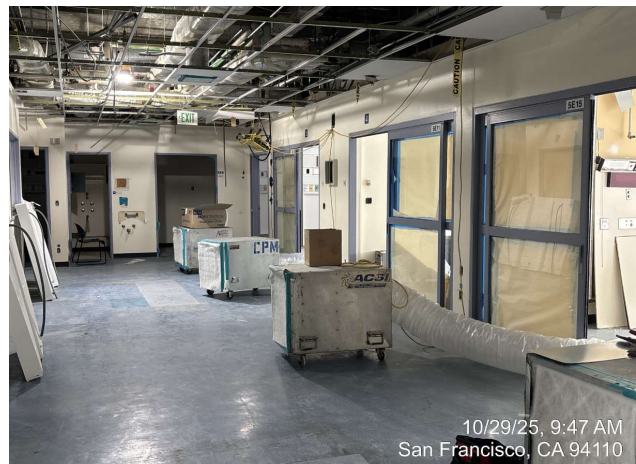
5E Temporary Construction Barriers and Infection Control Barriers
