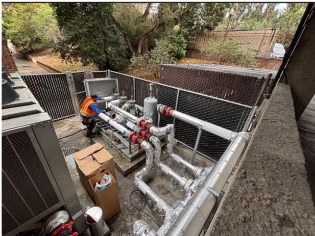
Installation of insulation at hydronic pumps
