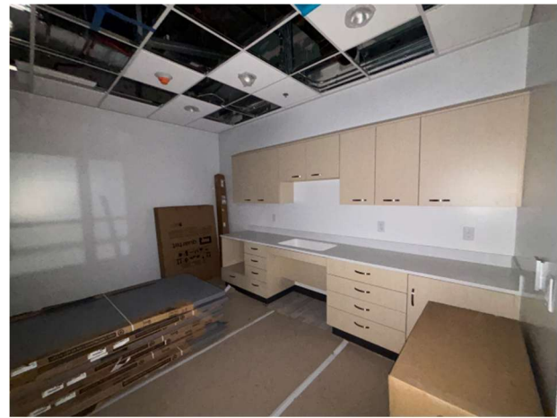
Casework Installation at Breakroom
