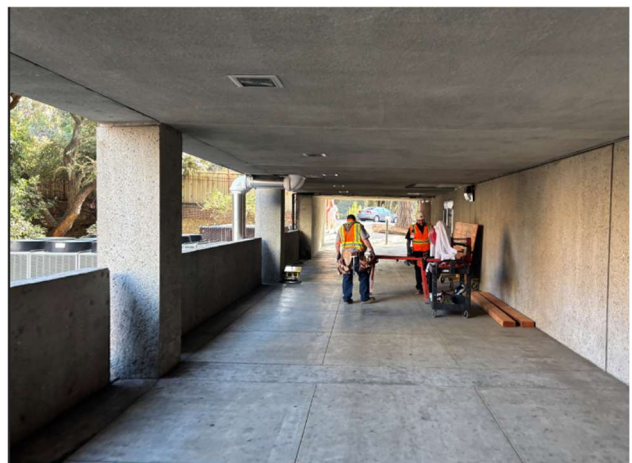
Repaired ceiling at breezeway after installation of piping inside ceiling plenum
