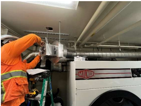
Installing control switch on booster fan in laundry room
