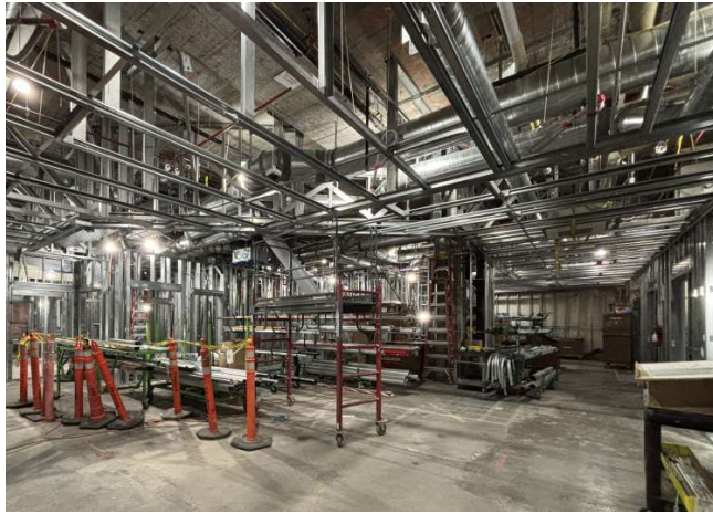
Framing and Drywall Installation West Corridor
