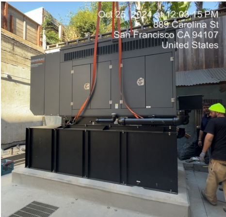
Generator installation at Station 37
